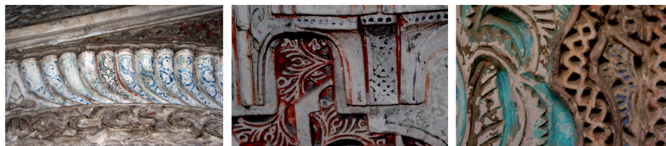
Fig. 1. Polychrome residues in medieval plasterwork. Left: royal chamber of Santo Domingo, Granada. Center: the oratory in the Madrasa, Granada. Right: royal Alcazar of Seville.
